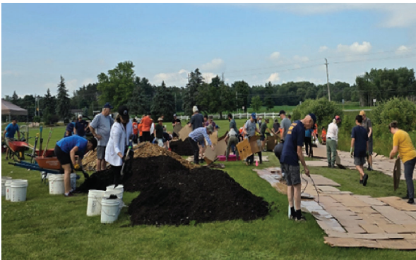
Site preparation for the "Little Forest" in Uxbridge
